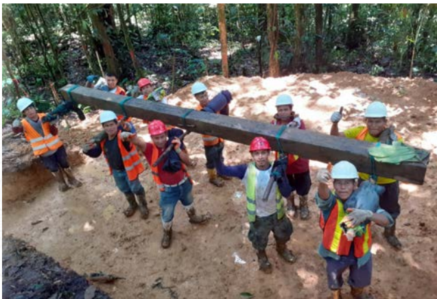
Figure 1. The first beams used to stabilize the drill rig arriving at a platform.
