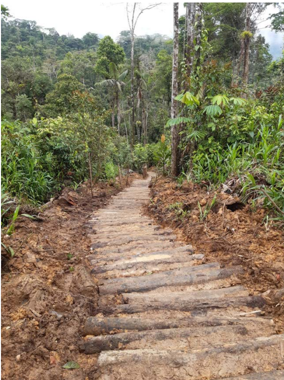
Figure 5. Log-paved paths mitigate the development of debilitating mud and also prevent erosion. The logs are all cut from fallen and dead standing trees.
