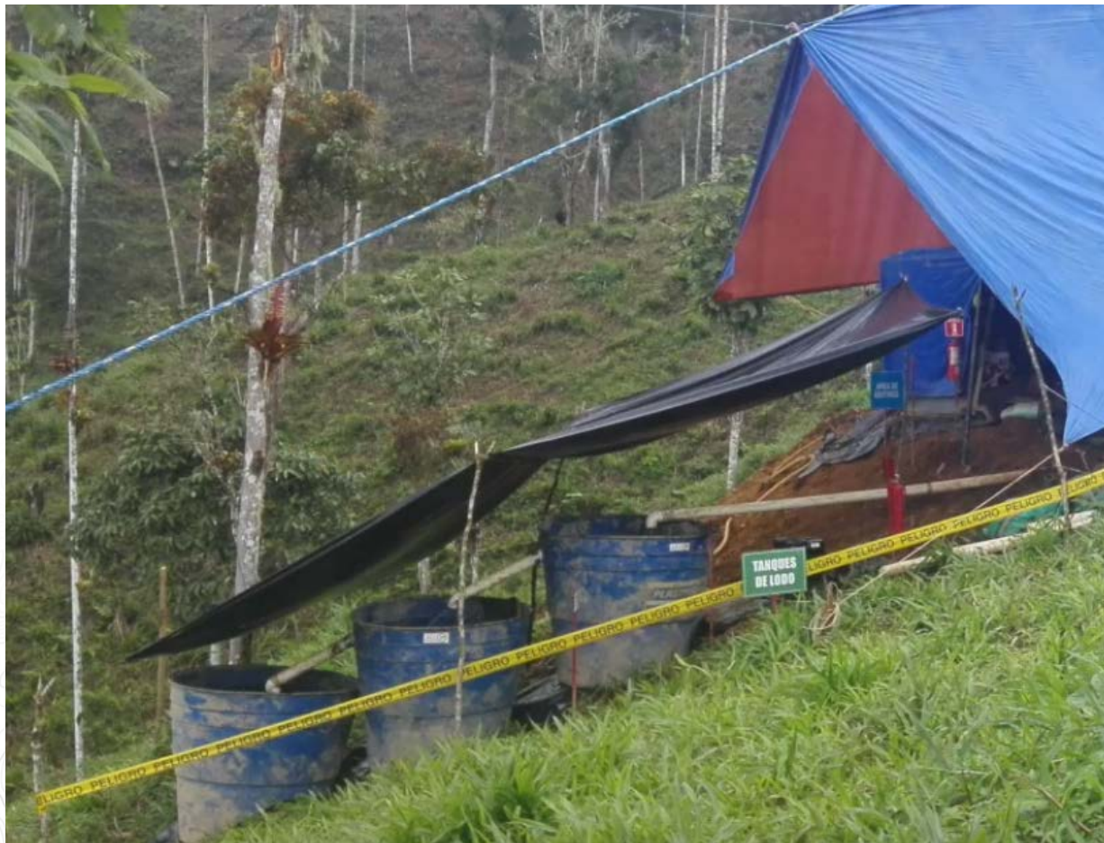
Figure 5. The blue tanks are settling tanks in which mud and rock powder from the drill hole settles and the clean water is recycled back down the drill hole.
