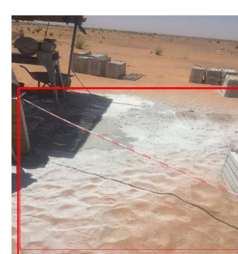
Fig 5 Soil pollution during core cutting.
