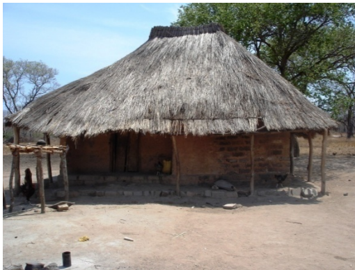
Plate 6.4 Mud-brick House with Grass Thatch
