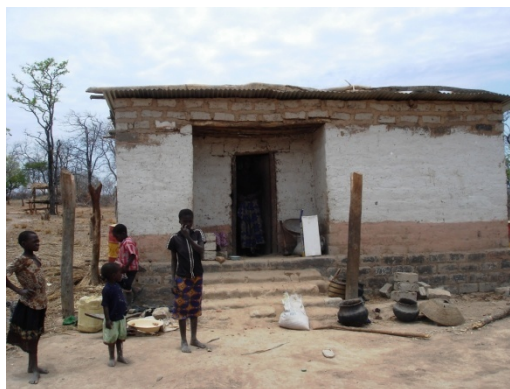
Plate 6.5 Mud-brick House with Iron Sheet Roof
