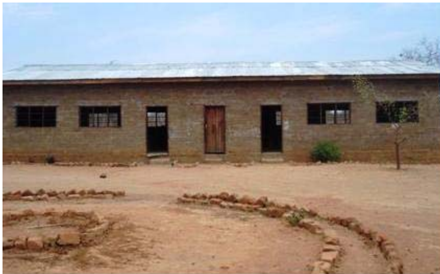
Plate 6.11 Classroom Block at Dibwi Community School
