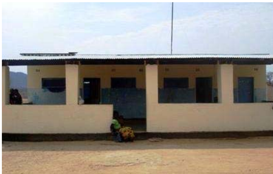
Plate 6.12 Manchama Rural Health Centre
