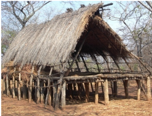
Plate 6.3 Pole and Grass Storage Shelter
